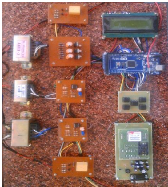
Fig. 2(a) Hardware Implementation
