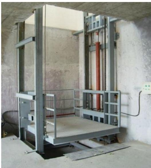
Fig(1): Hydraulic Elevator
